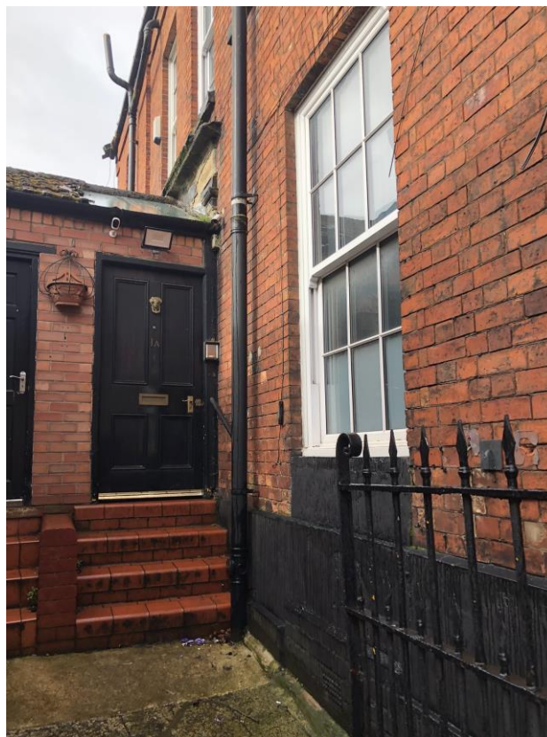
Figure 3. Entrance to the property from a personnel gate off Cavendish Road.
