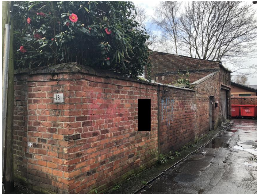
Figure 7. Rear boundary wall of applicant site in relation to rear alleyway.
