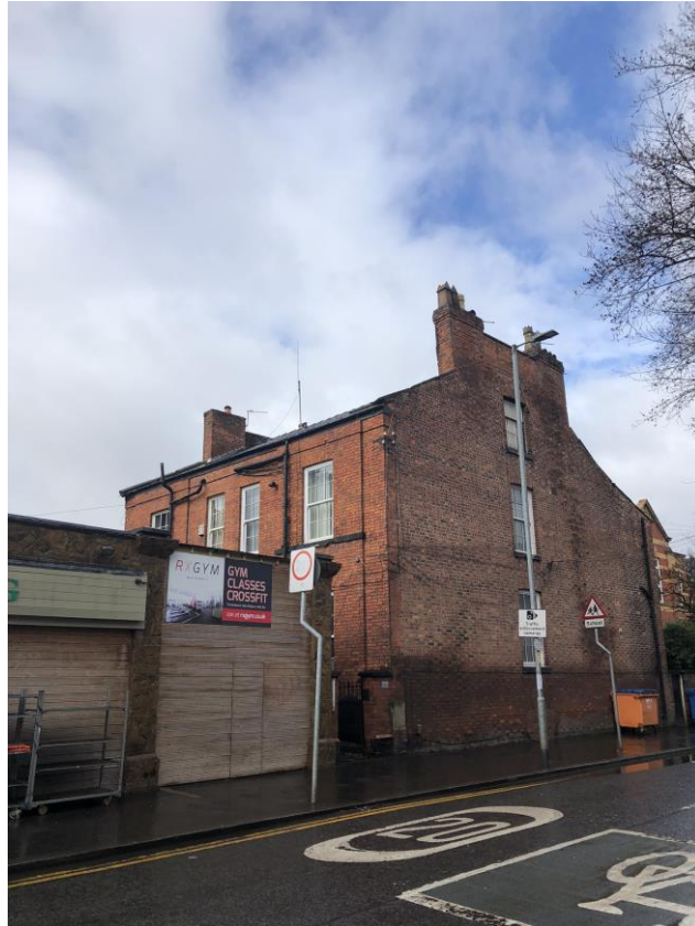
Figure 4. Primary view of the property as seen from Cavendish Road.
