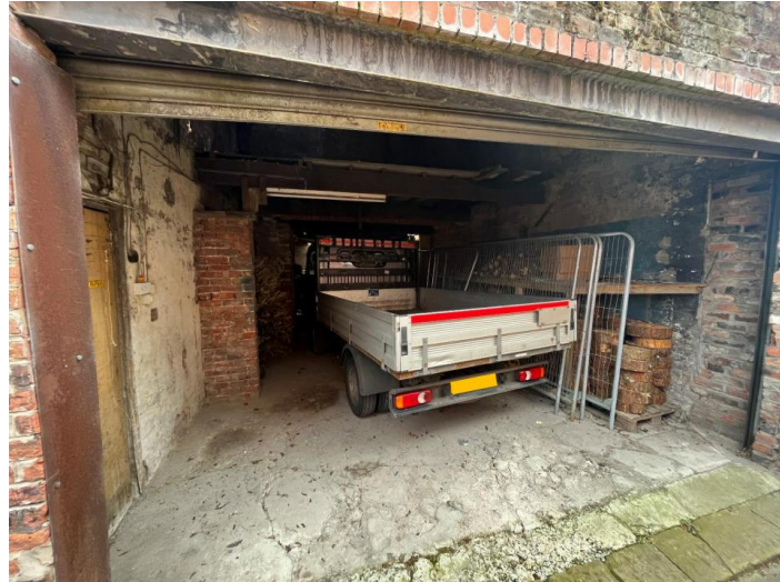
Figure 28. Garage at the end of the alleyway used for parking purposes by a neighbouring property
