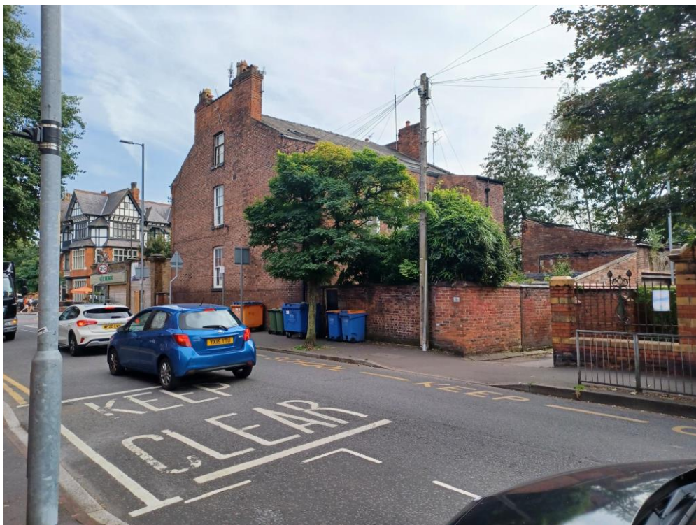
Figure 5. Rear view of the property as seen from Cavendish Road.
